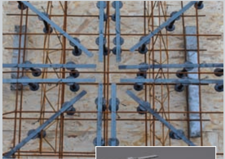
Figure 2 - Placement of Sheartech ® rails
