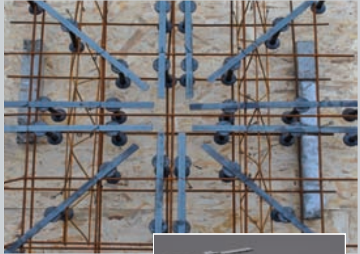
Figure 2 - Placement of Sheartech® rails
