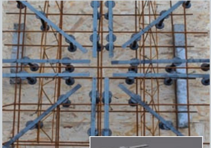
**Figure 2 - Placement of Sheartech® rails**
